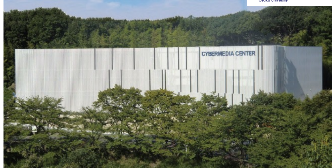
IT core as data center
