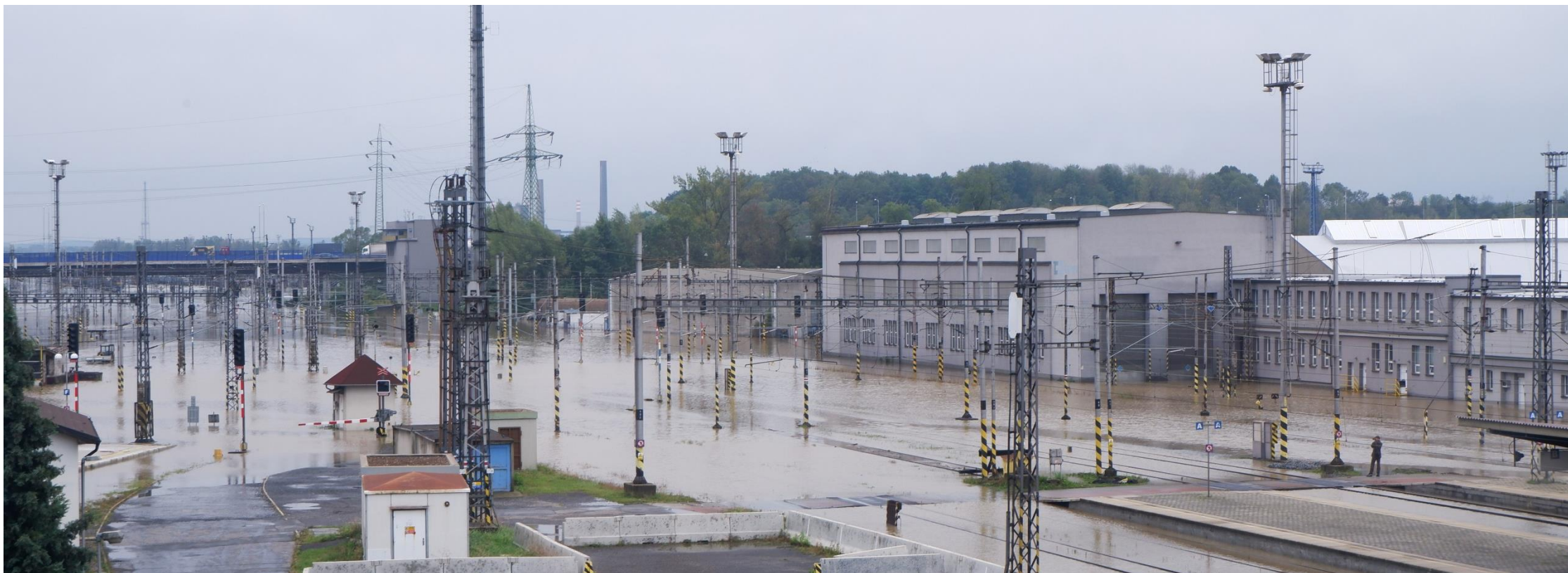
Flooded main railway station in Ostrava, Czech Republic
