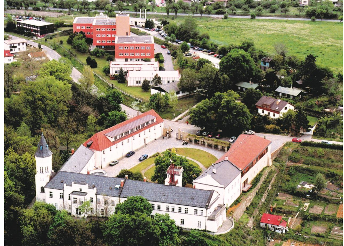
CHMI headquarters at Prague
